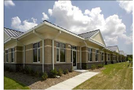
McComas Way Office Building, Virginia Beach, VA
