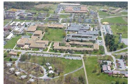
Building 802 Renovations, Woodrow Wilson Rehabilitation Center, Fishersville, VA
